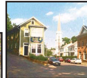
HISTORIC ARCHITECTURE MAIN STREET
